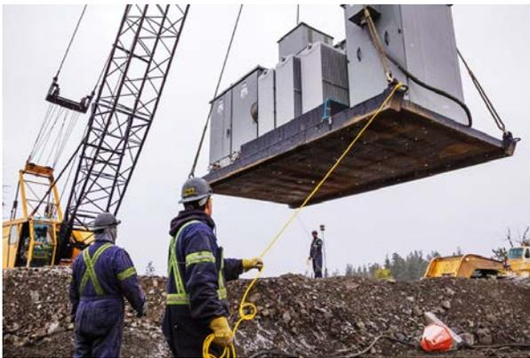
When sites are not accessible with a trailered unit, IMG substations are assembled on a rigid, steel skid typically consisting of 8x6" tubing skid, point-of-connection for tow/lift hooks, grated floor for non-skid, and oil-containment where required. Outdoor-type enclosures are used for Incoming & Outgoing sections to protect equipment from environmental elements.
