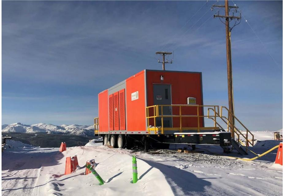
Typically, they consist of an Incoming Section, Transformer Section and Outgoing section. Outgoing section can have 2-3 feeder units that distribute power to various site, electrical equipment.
